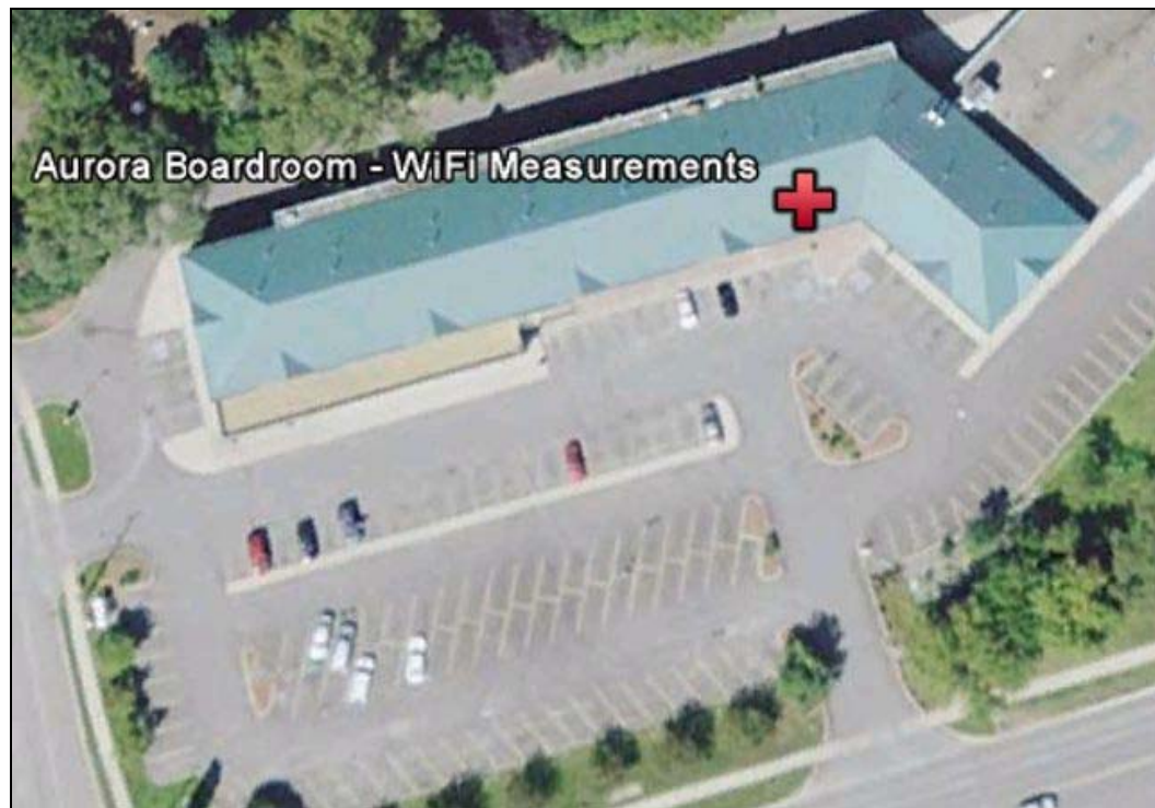
Figure 3 – Aerial view of the measurement location in Aurora, Ontario
