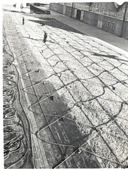
Boom defence net laid out at Esquimalt, British Columbia
