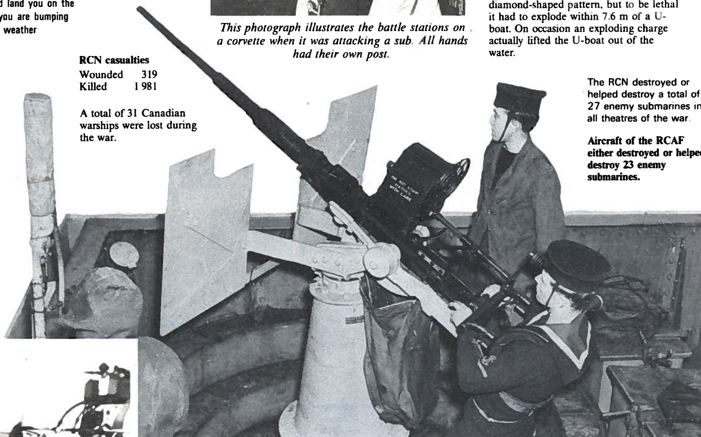
Each corvette was armed with two 40 mm orlikons which were used as anti-aircraft guns and as a weapon against personnel on enemy ships if the gun could be depressed enough.
